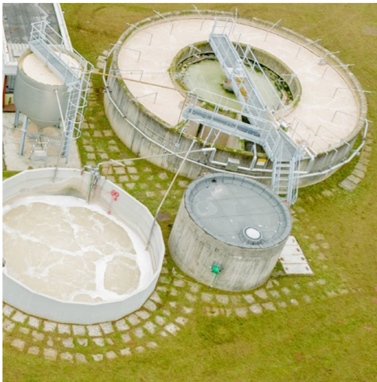
Wastewater treatment plant Origgio Site
